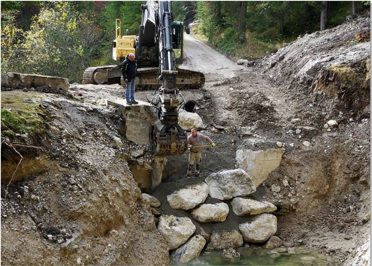
Fig 6: Forming the outflow of the spring pot. Photo: R. Seebacher
