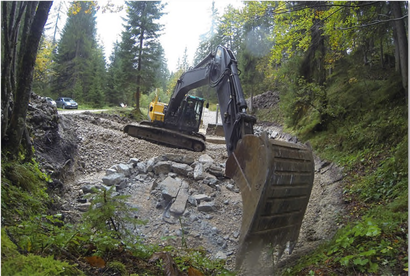
Fig 4: Start of the deconstruction work. Photo: R. Seebacher
